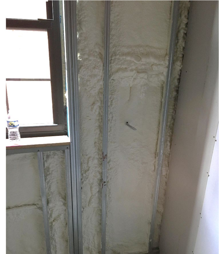
Spray foam fills the gap
